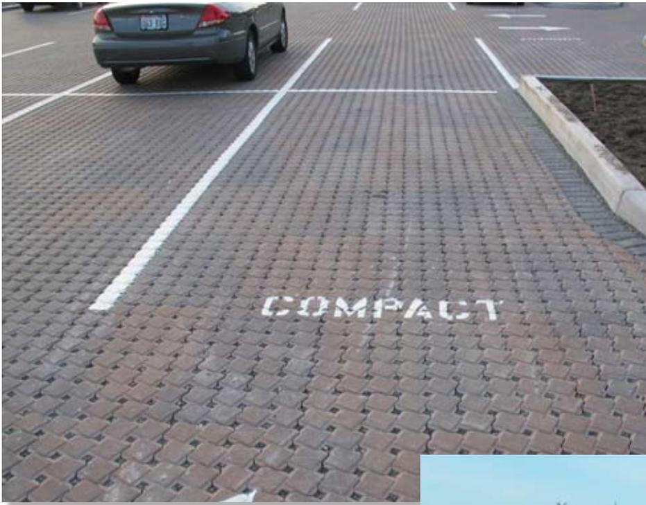
The sandy loam subgrade provides filtering of runoff, capturing pollutants typical of an automobile parking lot.
